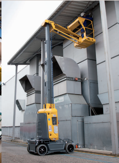
MAINTENANCE AND OUTSIDE INFRASTRUCTURE CHANGES (lighting, signage, repairs, etc.)
